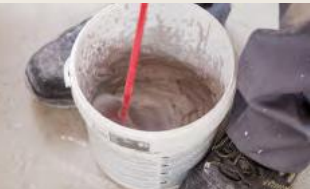
PREPARE THE GROUT ·
