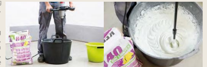
PREPARE THE ADHESIVE CEMENT
