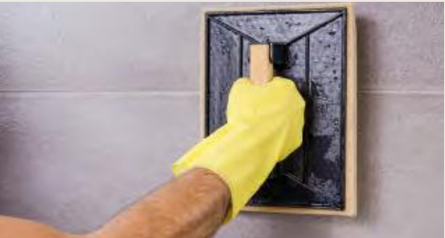
REMOVE ANY LEFTOVER GROUT AND OTHER DIRT
