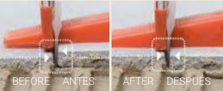
1. Insert the wedges in the clip slot, making sure you don't pass the breakpoint.
