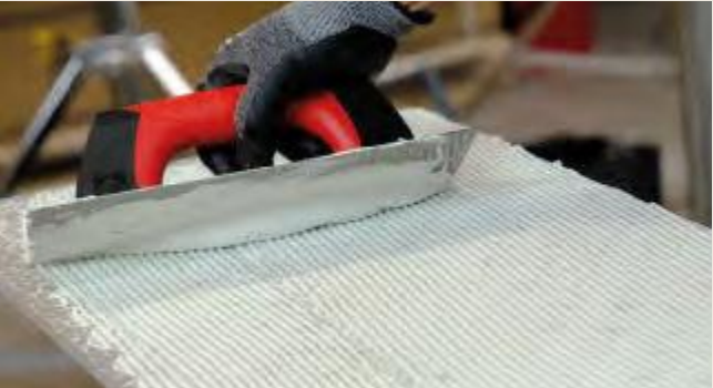
MAKE SURE THE THICKNESS OF THE LAYER OF ADHESIVE CEMENT IS UNIFORM
