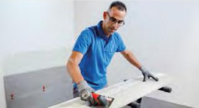
SPREAD THE ADHESIVE CEMENT WITH A TOOTHED TROWEL ON THE TILE ·
