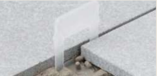
1. After spreading the adhesive cement, insert the clips underneath the tiles on all four sides.
