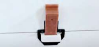
2. For large tiles, use more clips on each side.
