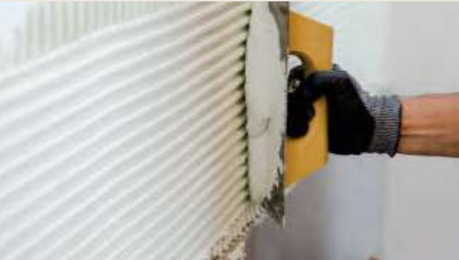
MAKE SURE THE THICKNESS OF THE LAYER OF ADHESIVE CEMENT IS UNIFORM
