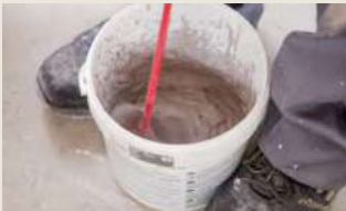
PREPARE THE GROUT ·
