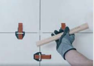
2. For large tiles, use more clips on each side.
