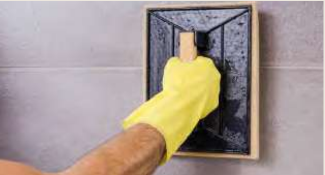
REMOVE ANY LEFTOVER GROUT AND OTHER DIRT
