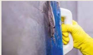
USE A GROUT TROWEL TO AFFIX THE MATERIAL ·
