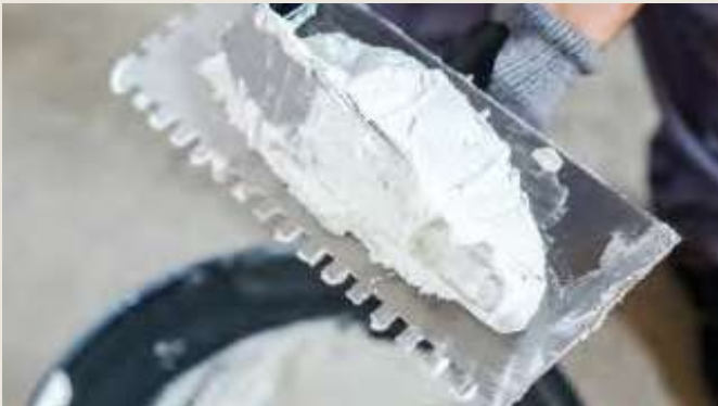
SPREAD THE ADHESIVE CEMENT WITH A TOOTHED TROWEL
