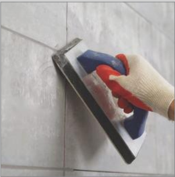
Joint Grouting
