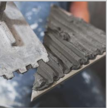
Cement Laying On Tile
