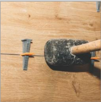
Remove Wedges Ones It Dry
