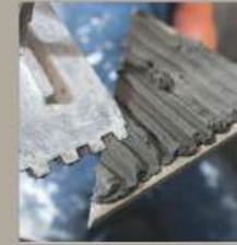
Cement Laying On Tile
