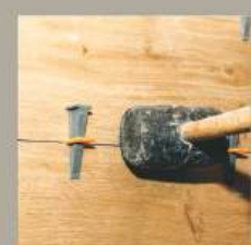
Remove Wedges Once it Dry
