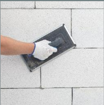
Joint Grouting
