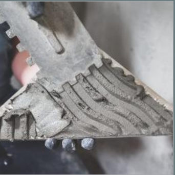
Cement laying on tile
