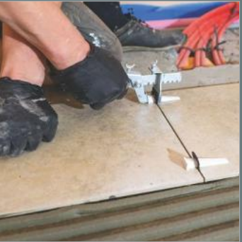
Levelling Wedges
