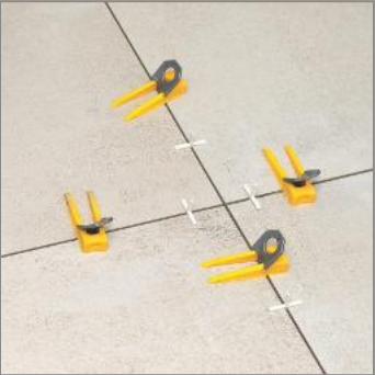
After Lavelling Process Leave Int For 8-10 Hrs.
