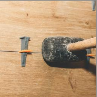
Remove Wedges Ones It Dry
