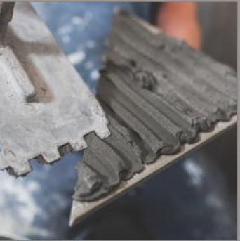
Cement Laying On Tile
