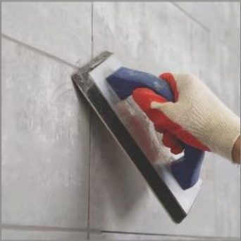
Joint Grouting
