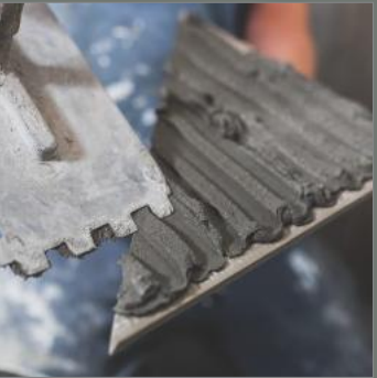
Cement Laying On Tile
