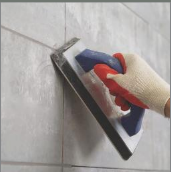
Joint Grouting
