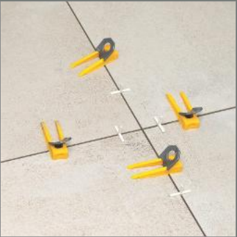
After Lavelling Process Leave Int For 8-10 Hrs.
