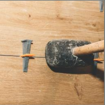
Remove Wedges Ones It Dry
