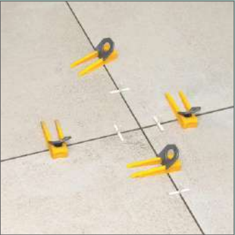
After Lavelling Process Leave Int For 8-10 Hrs.
