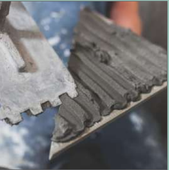
Cement Laying On Tile
