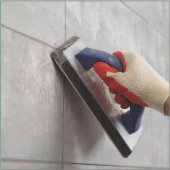
Joint Grouting
