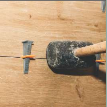
Remove Wedges Ones It Dry
