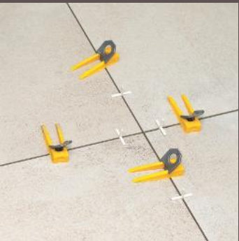
After Lavelling Process Leave Int For 8-10 Hrs.
