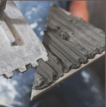
Cement Laying On Tile
