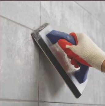
Joint Grouting
