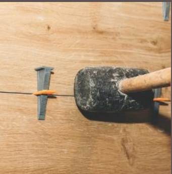
Remove Wedges Ones It Dry
